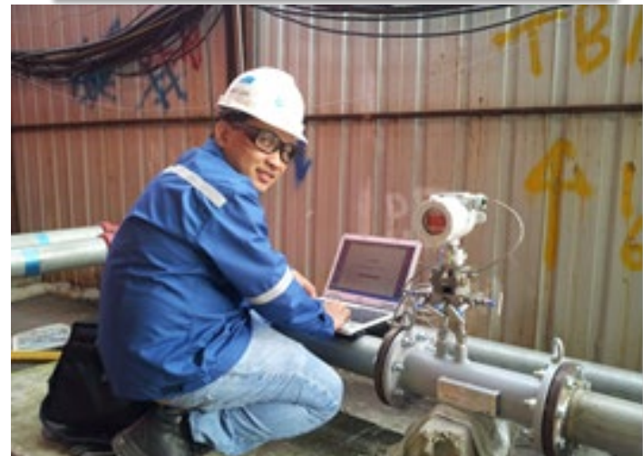
DP Cone Flow Meter commissioning
