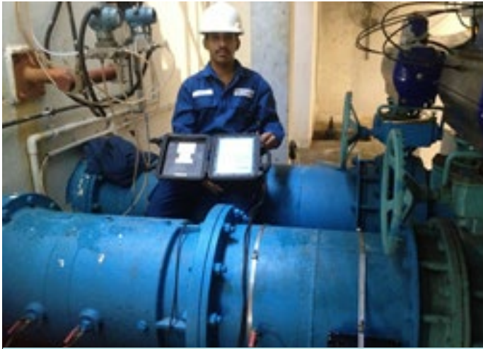
Flow Survey at Woodleigh Waterworks
