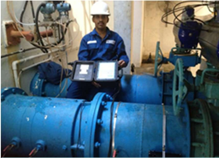
Flow Survey at Woodleigh Waterworks
