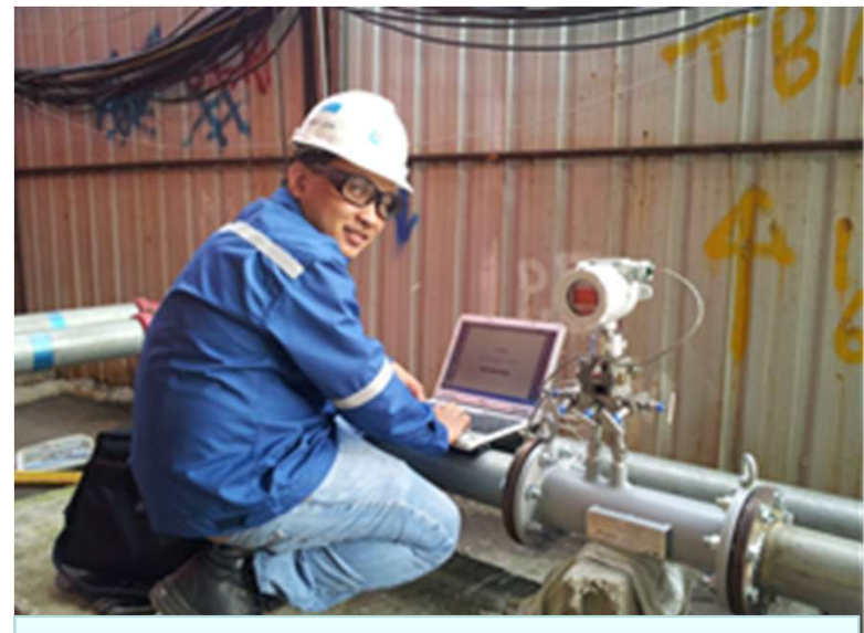
DP Cone Flow Meter commissioning
